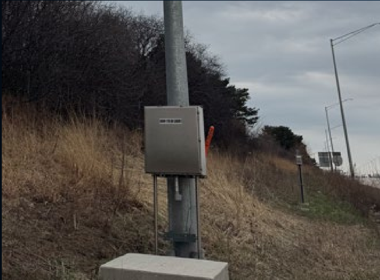
ITS Enclosure with Type B Concrete Foundation
