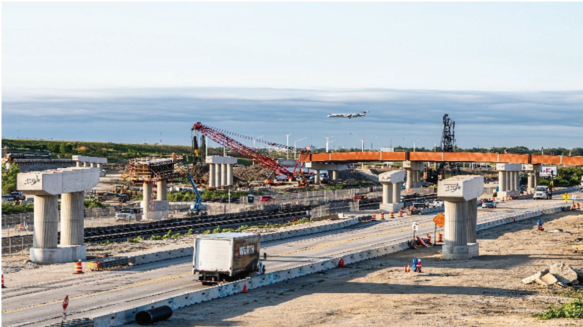
I-490/IL 390 Interchange construction near Bensenville.
