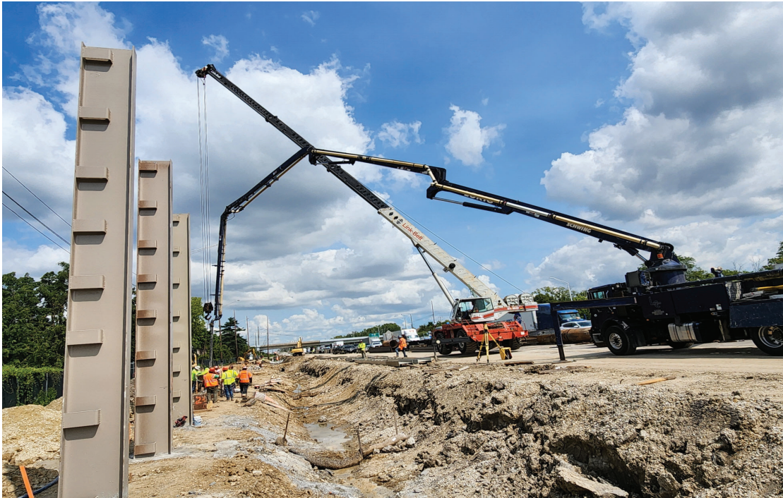
I-290/I-88 Interchange Project at I-294, facing north near Elmhurst.
