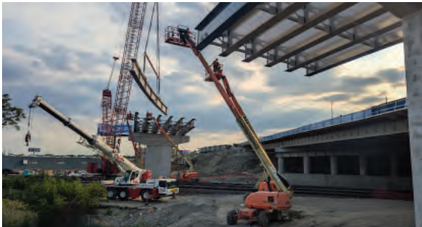
Beam placement for the I-490/I-294 Interchange near Franklin Park.
