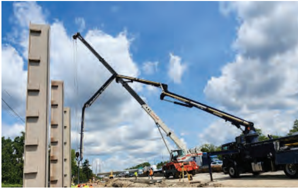
Noisewall construction continues along the Central Tri-State Tollway (I-294) near Westchester.
