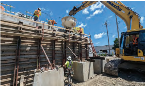
Bridge work continues in Bensenville near Grand Avenue.
