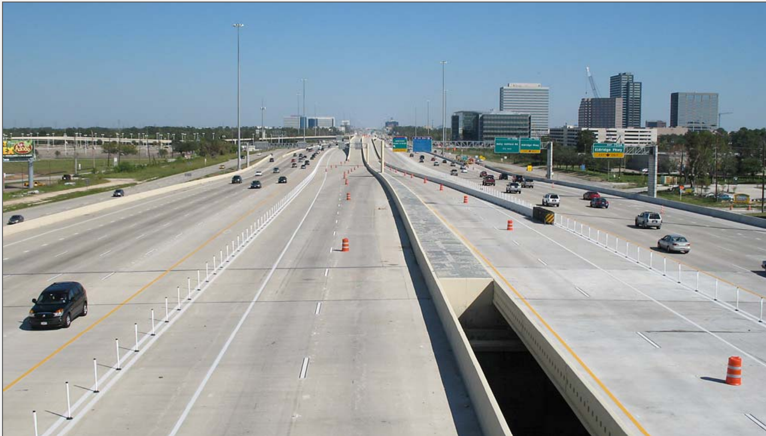
Katy Tollway Managed Lanes Houston, TX
