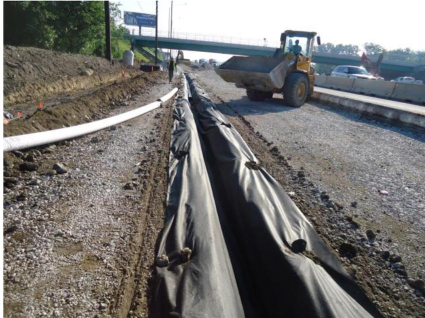
Pipe underdrain is being installed along I-57 for the new ramp from southbound Tri-State Tollway (I-294) to southbound I-57 (6/27/2013)
