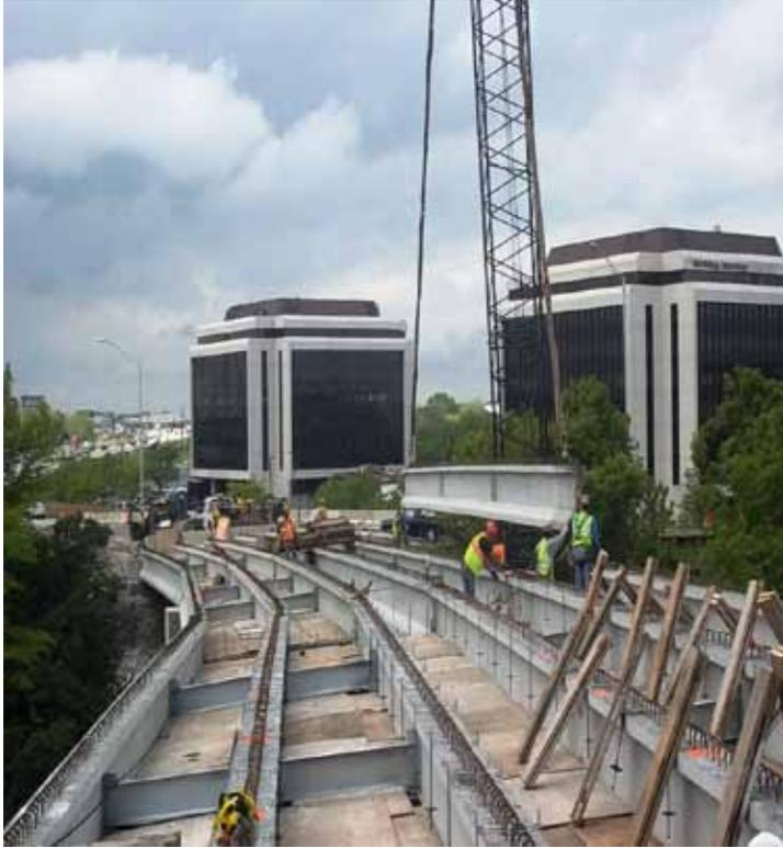
Crews install beams on the Tri-Level Bridge ramp structure from northbound Tri-State Tollway (I-294) to west-bound Jane Addams Memorial Tollway (I-90)
