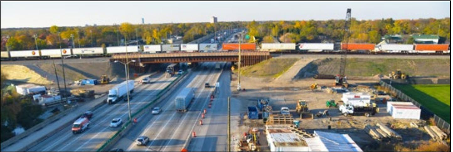
Working in coordination with the Burlington Northern Santa Fe Railway, the Illinois Tollway has completed construction of the temporary bridge – or shoofly bridge – to allow for uninterrupted commuter rail and freight operations during reconstruction of the BNSF Bridge over the Central Tri-State Tollway (I-294).
