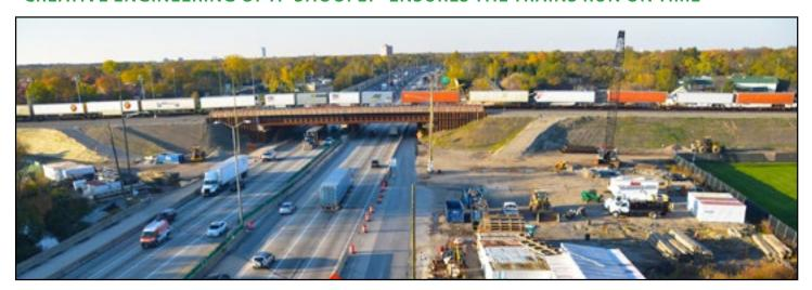
Working in coordination with the Burlington Northern Santa Fe Railway, the Illinois Tollway has completed construction of the temporary bridge – or shoofly bridge – to allow for uninterrupted commuter rail and freight operations during reconstruction of the BNSF Bridge over the Central Tri-State Tollway (I-294).
