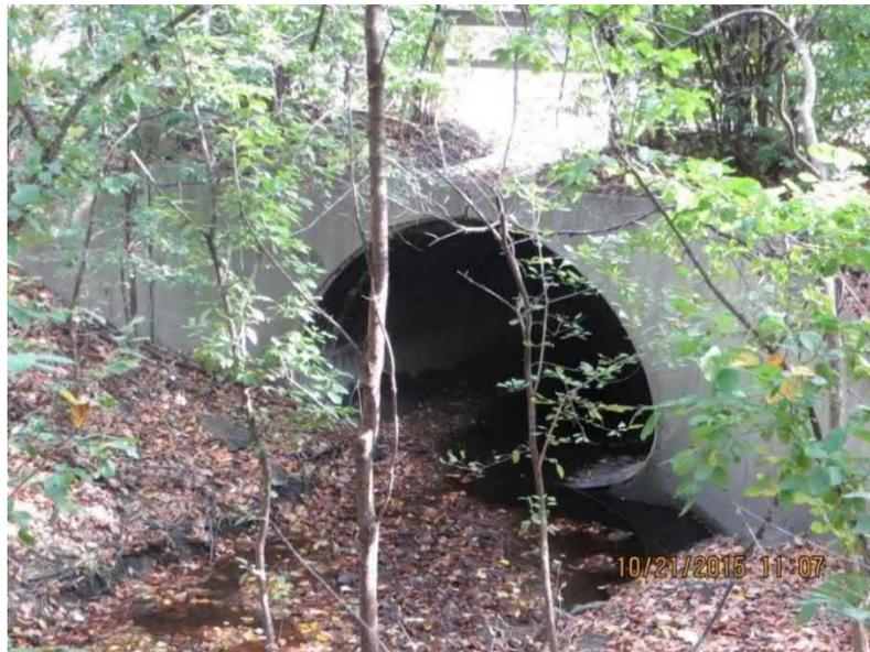
**Figure 7: 11.6' (W) x 7.33' (H) Arch CMP Culvert under Creek Drive**
