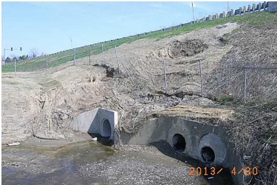
**Figure 15: Erosion of the Cermak Road Bridge along I-294**
