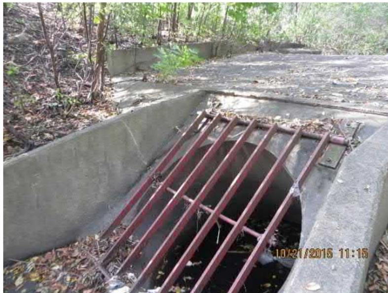
**Figure 9: Concrete Grate Structure, downstream of Creek Drive**
