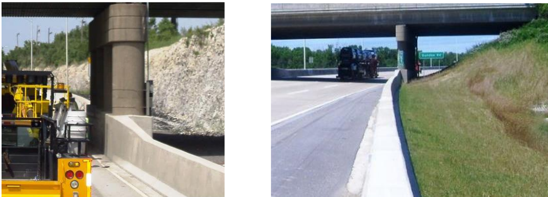
Figure 13.2a Concrete Shoulder Barrier Transition
