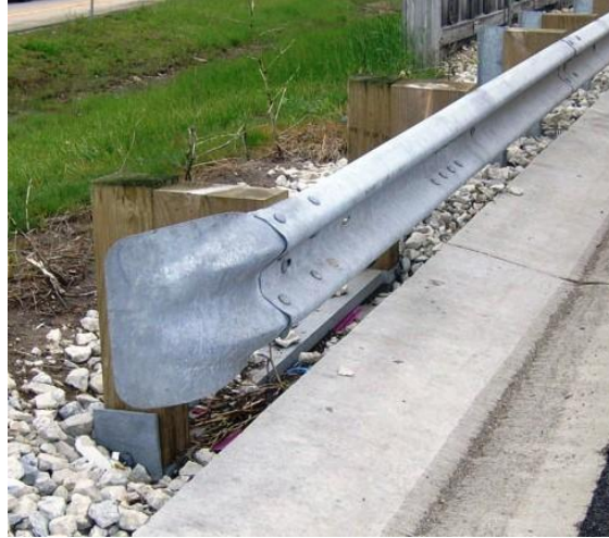
Figure 10.5.1b Traffic Barrier Terminal Type T2 – Without Gutter
