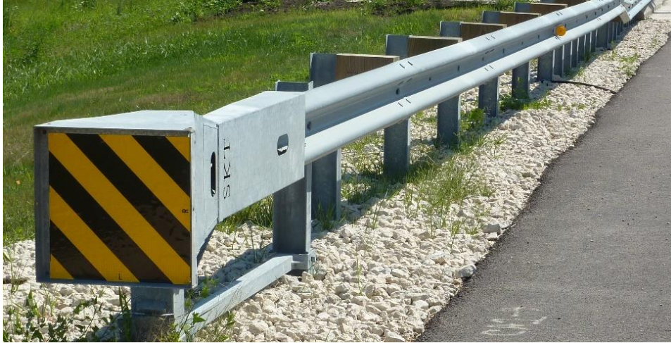
Figure 10.3.2a Traffic Barrier Terminal Type T1-A (Special)
