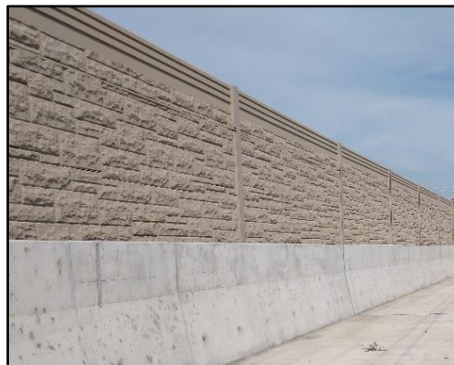
Figure 3.8b Noise Abatement Wall Attached to Parapet (Structures)
