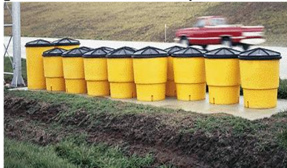
Figure 11.2 Sand Module Impact Attenuator
