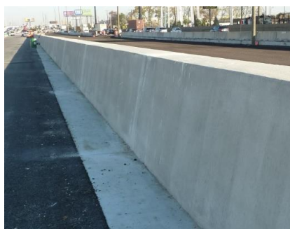
Figure 13.3 Concrete Barrier Double Face
