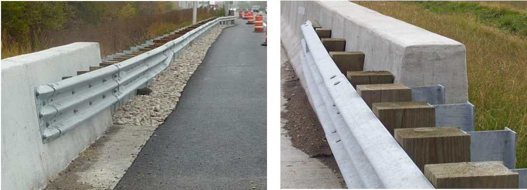
Figure 10.6.2 Traffic Barrier Terminal Type T6B
