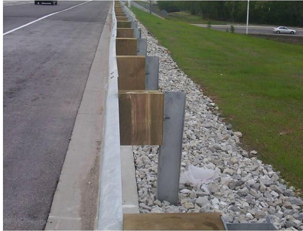
Figure 9.0 Midwest Guardrail System
