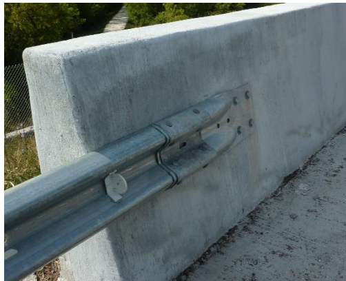
Figure 10.4.2 Traffic Barrier Terminal Type T10
