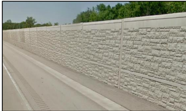
Figure 3.8b Noise Abatement Wall Attached to Parapet (Structures)
