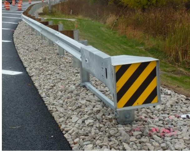
Figure 10.3.1b Traffic Barrier Terminal Type T1 (Special) - With Modified Gutter
