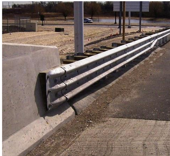
Figure 10.6.1 Traffic Barrier Terminal Type T6
