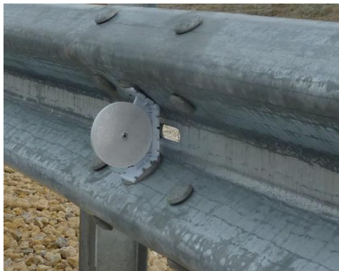
Figure 9.9 Guardrail Reflector
