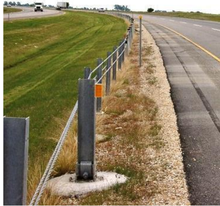
Figure 12.0 Cable Median Barrier
