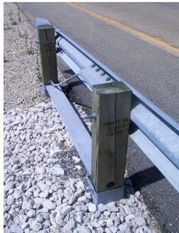
Figure 10.5.1b Traffic Barrier Terminal Type T2 – Without Gutter
