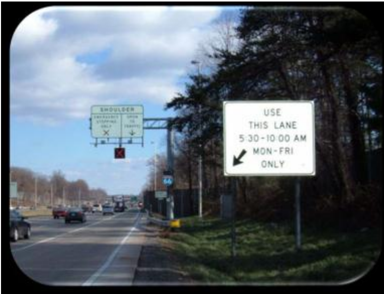
Source: FHWA I-66 in Virginia
