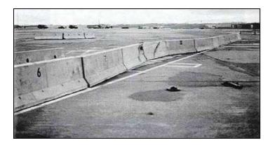
Individual barrier units set atop pavement which are attached together by a constrained pin and loop type connection.
