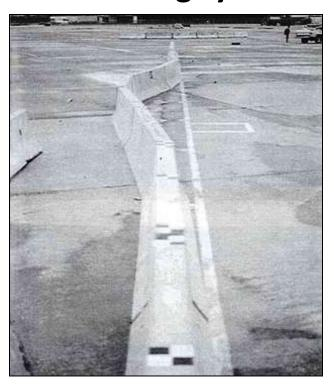
Free-standing TCB placement consists of the end barrier units being anchored into pavement or deck.
