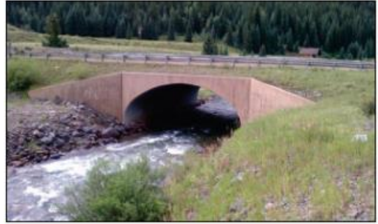
Figure 1 - Example of soft-bottom, or open, culvert. Image from FHWA (2012B). Soft-bottomed culverts reduce impacts to stream beds, allow for natural bed movement and minimize impacts to WOUS.
