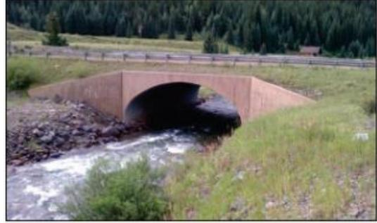
**Figure 1** - Example of soft-bottom, or open, culvert. Image from FHWA (2012B). Soft-bottomed culverts reduce impacts to stream beds, allow for natural bed movement and minimize impacts to WOUS.
