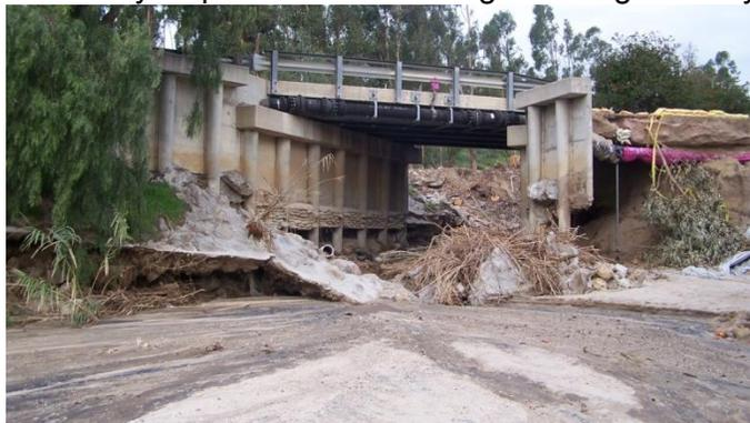
**Figure 3** - Example of long-term degradation at a historic bridge. Image from Caltrans, Division of Maintenance ([www.dot.ca.gov](http://www.dot.ca.gov)).
