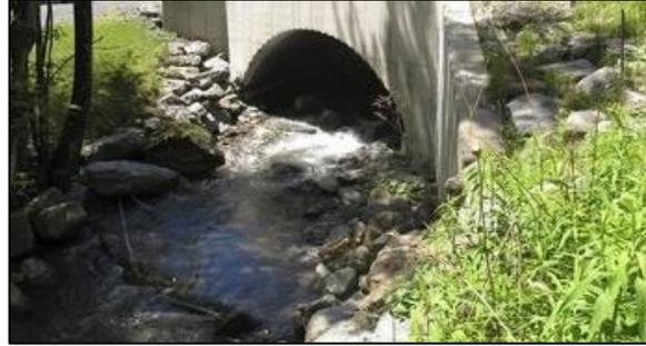
**Figure 6** - Culvert on Crossett Brook, Danbury, CT. This is an example of downstream grade control that allows for fish passage. (AP photo).
