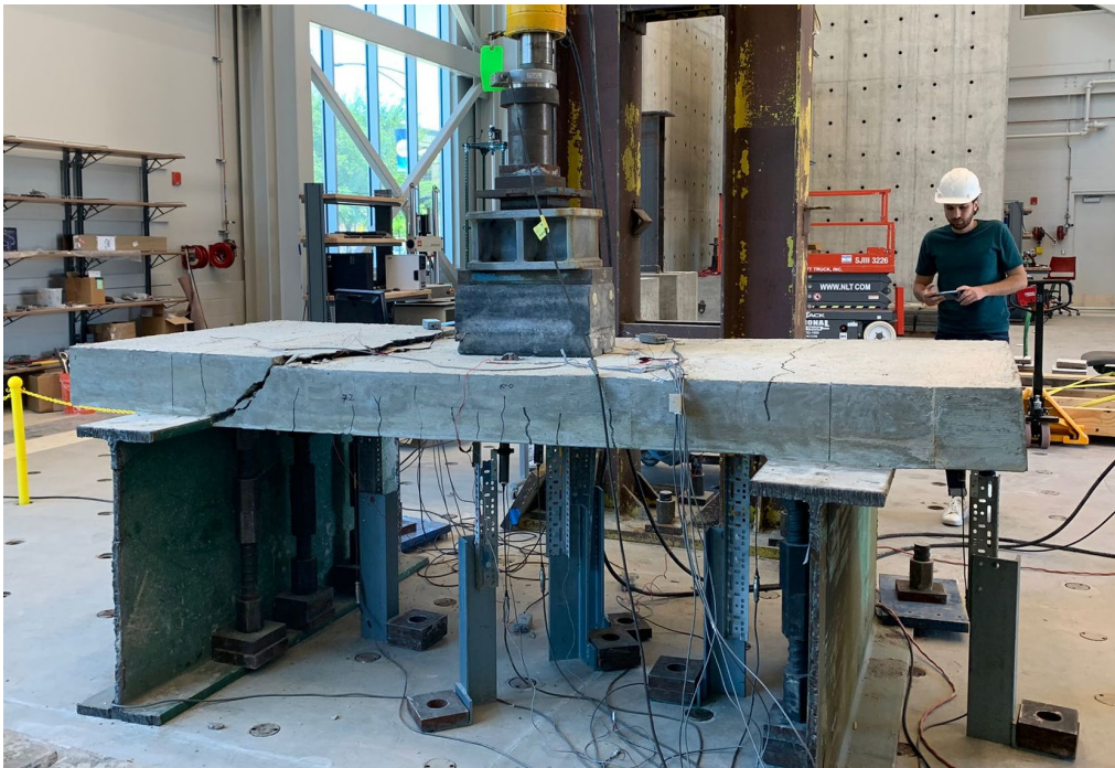
Figure 90: Mode of failure of bridge deck Prototype 4.
