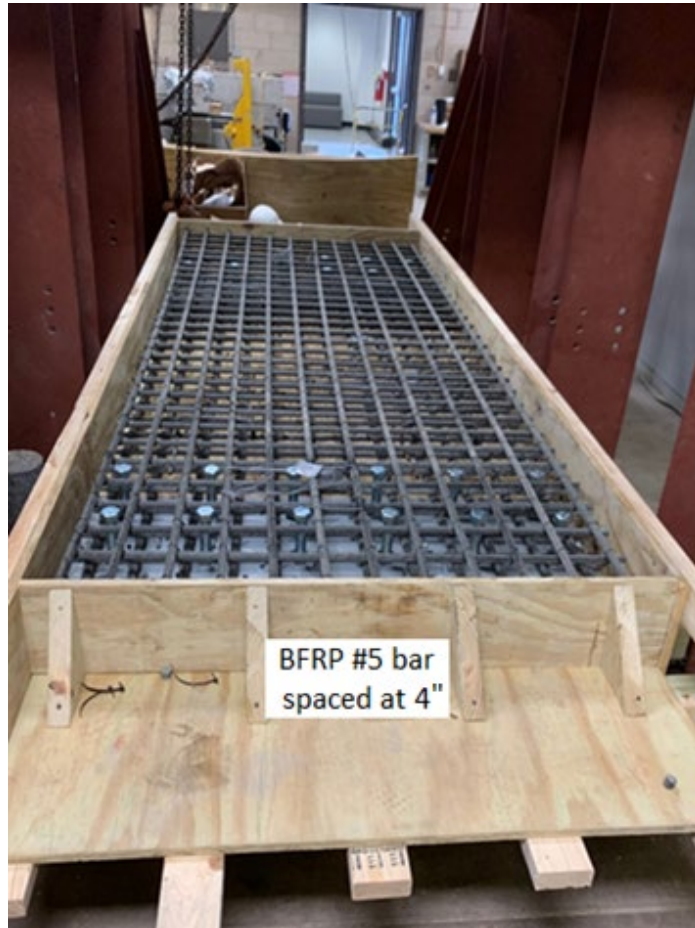
Figure 47: Single-span bridge deck slab before pouring the concrete.
