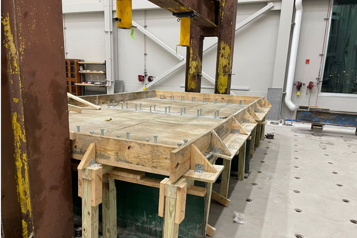
Figure 110: Formwork of two-span Prototype 6.
