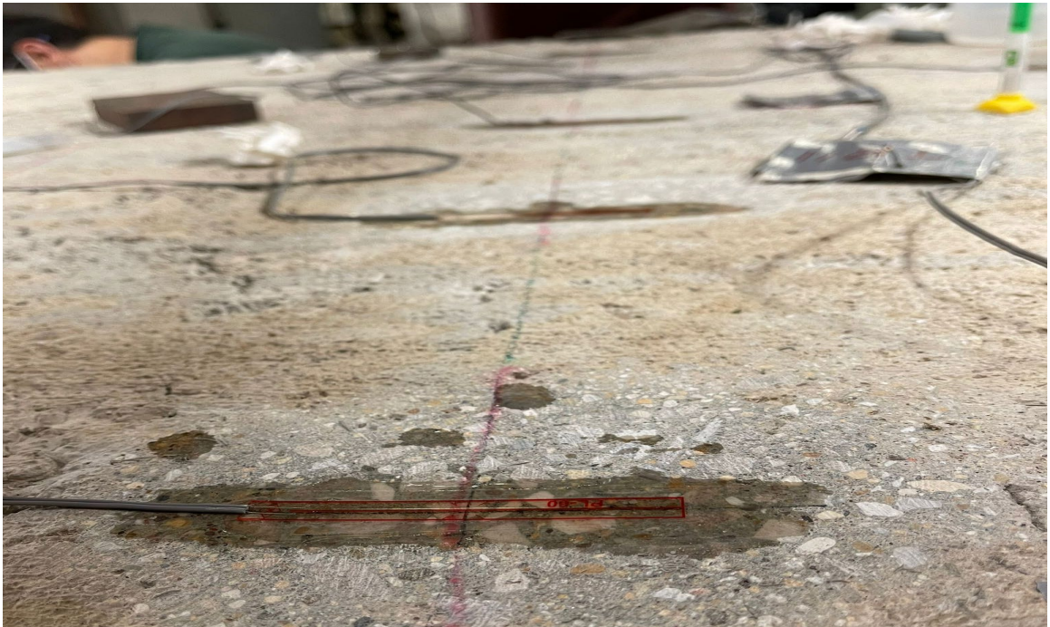
Figure 70: Concrete strain gauges, LVDT, and crack-meters installed on bridge deck Prototype 2.
