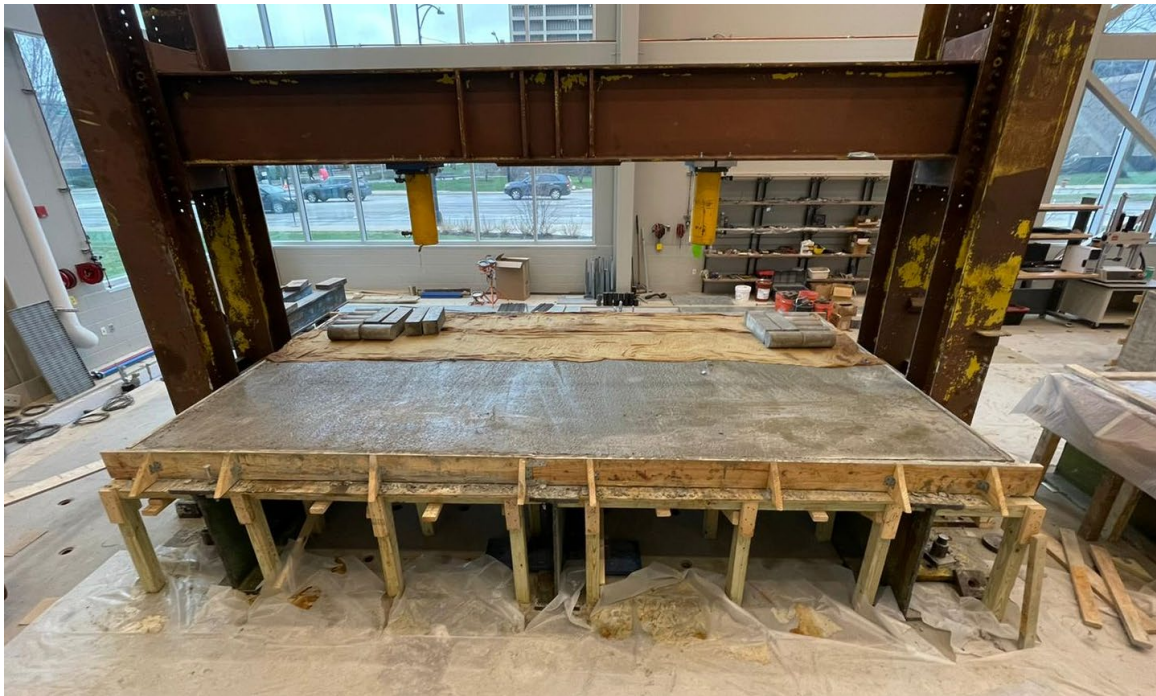
Figure 112: Cast of Concrete for the two-span bridge deck Prototype 6.
