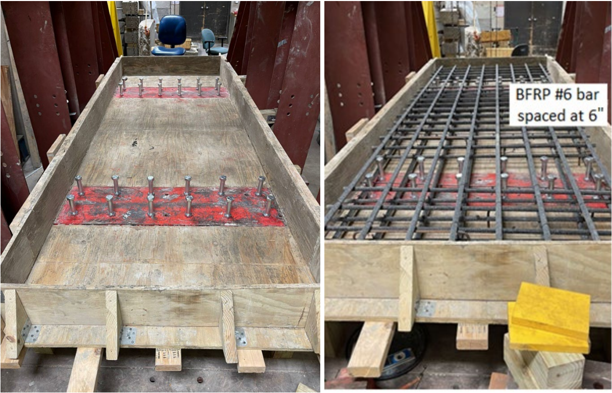
Figure 75: Formwork and BFRP reinforcement mesh of bridge deck Prototype 3.
