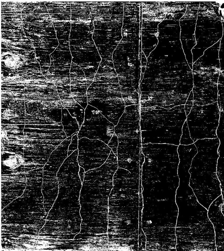
Figure 72: Crack mapping at the bottom midspan of bridge deck Prototype 2.
