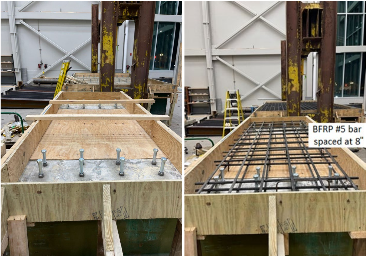
Figure 84: Formwork and BFRP reinforcement mesh of bridge deck Prototype 4.
