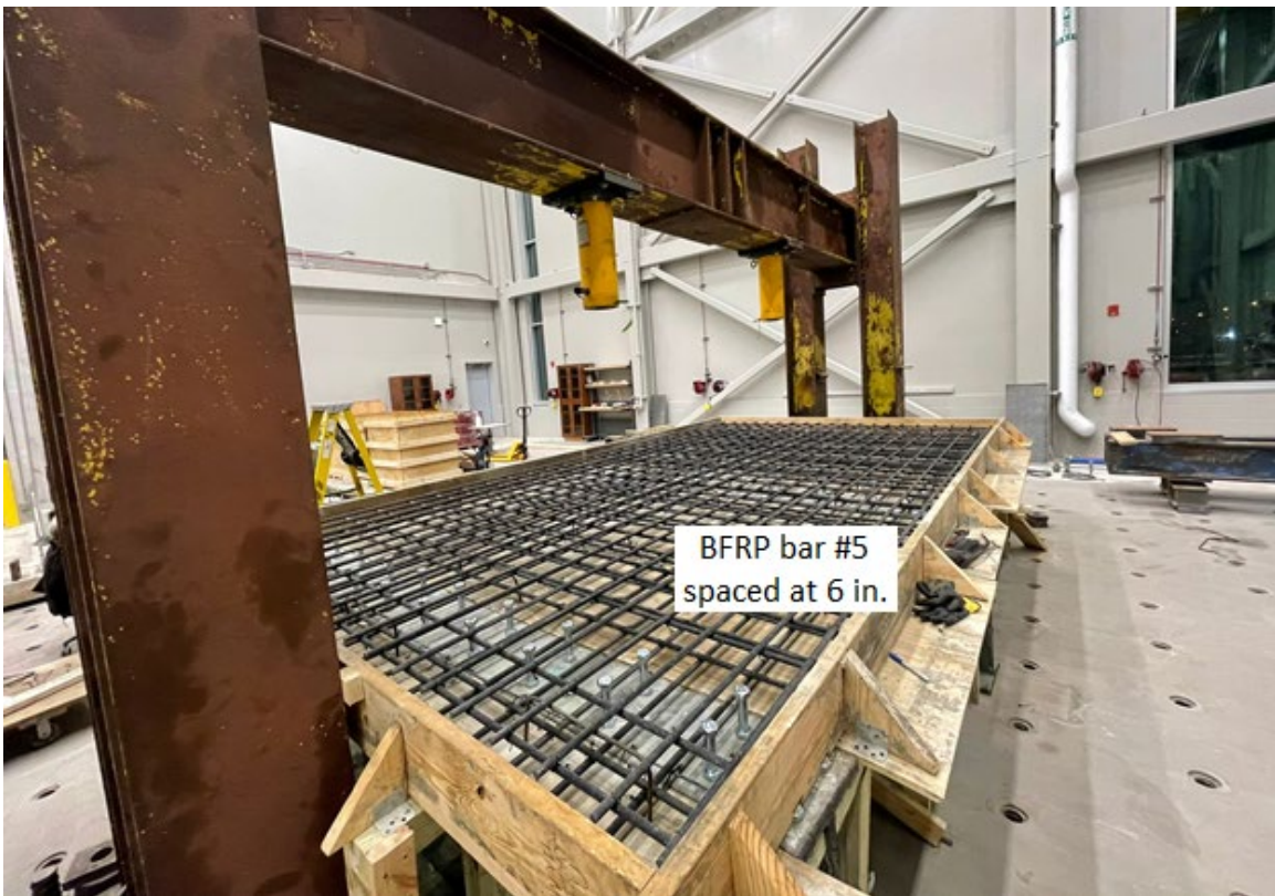
Figure 111: BFRP reinforcing bars in two-span Prototype 6.
