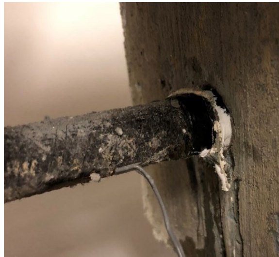
Figure 19: Slippage of BFRP bar from concrete.
