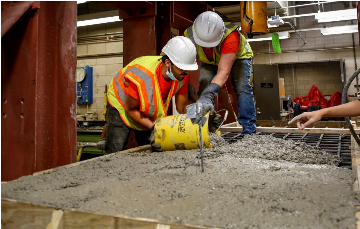
Figure 64: Single-span bridge deck Prototype 2 before and during the concrete pour.
