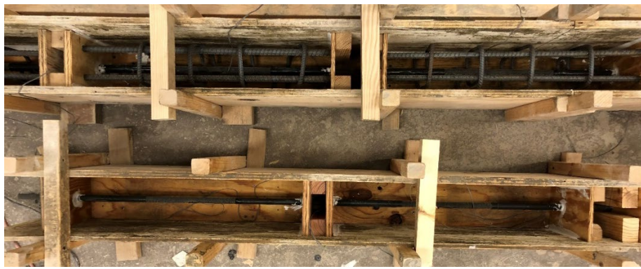
Figure 14: Hinged beam wood forms and testing setup.
