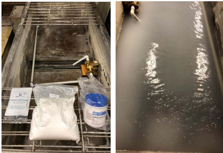
Figure 31: Alkaline solution tank with circulation.
