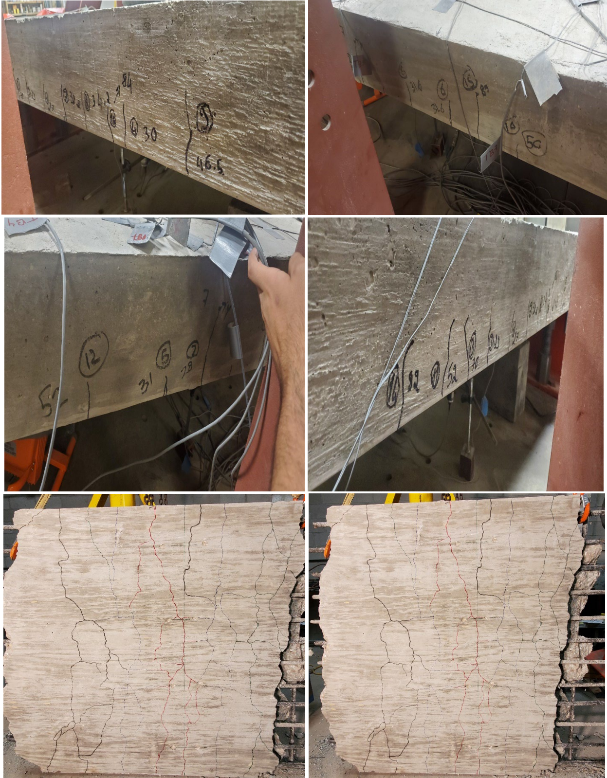
Figure 54: Crack mapping of the bottom face of bridge deck Prototype 1.
