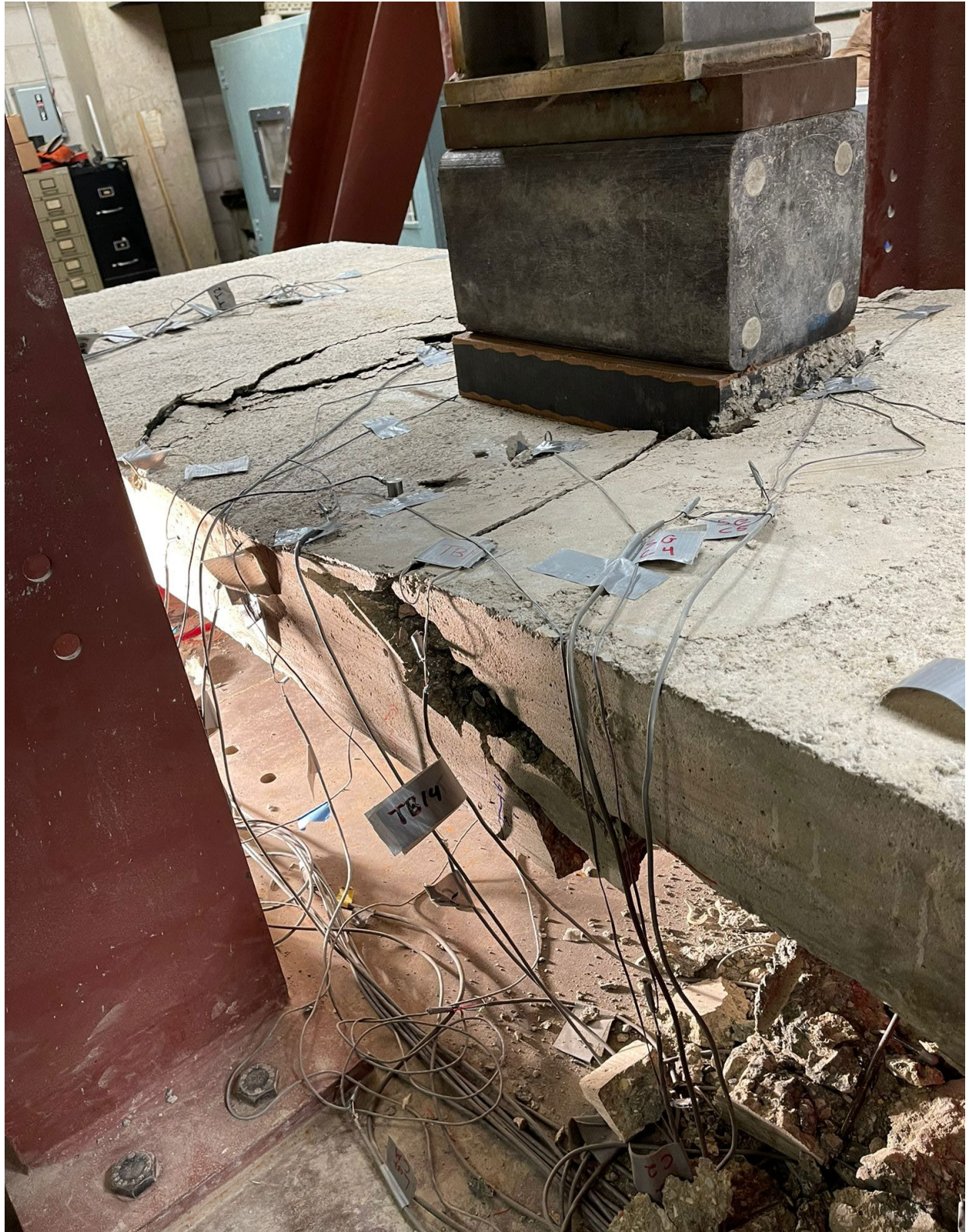
Figure 71: Failure mode of bridge deck Prototype 2.
