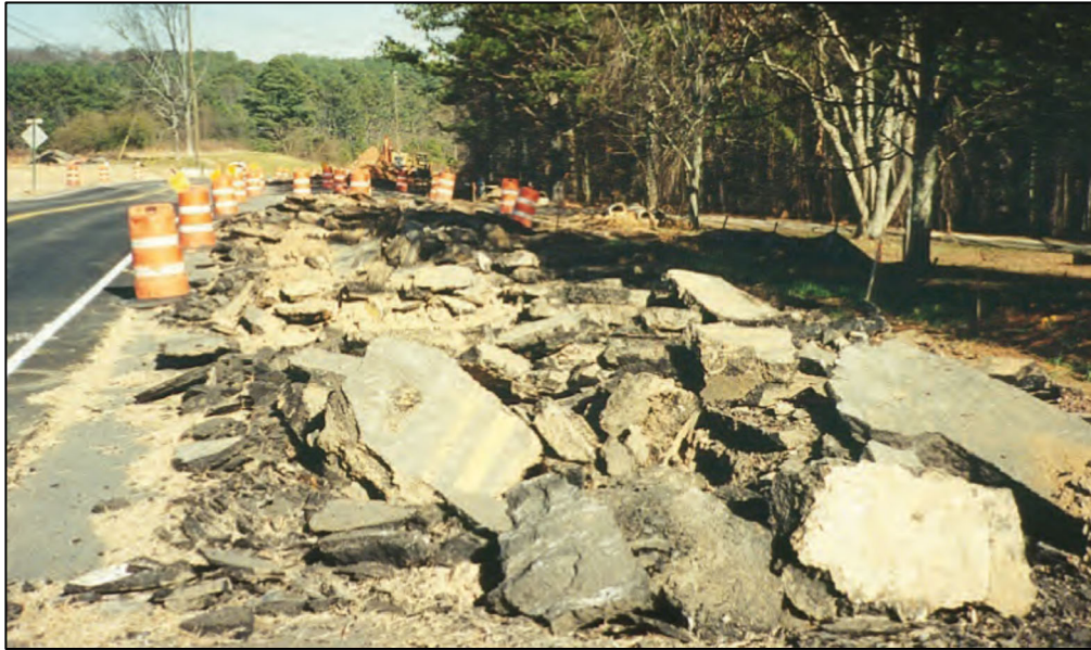
FIGURE 2. Road slabs produced from full-depth demolition (West, 2015).
