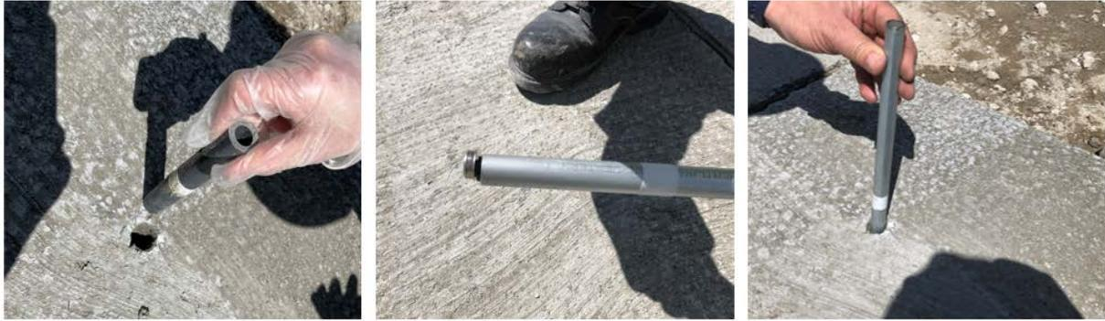
Figure 4-17. Installation of iButtons (L-R: removing plastic pipe after concrete hardened, placing iButton using magnetic stick, covering the space above iButton using the plastic pipe to form a seal)
