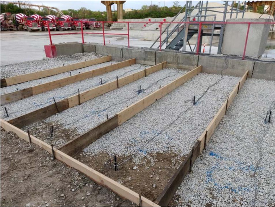
Figure 4-11. Strain gages and positioning chairs setup (photographed facing south)
