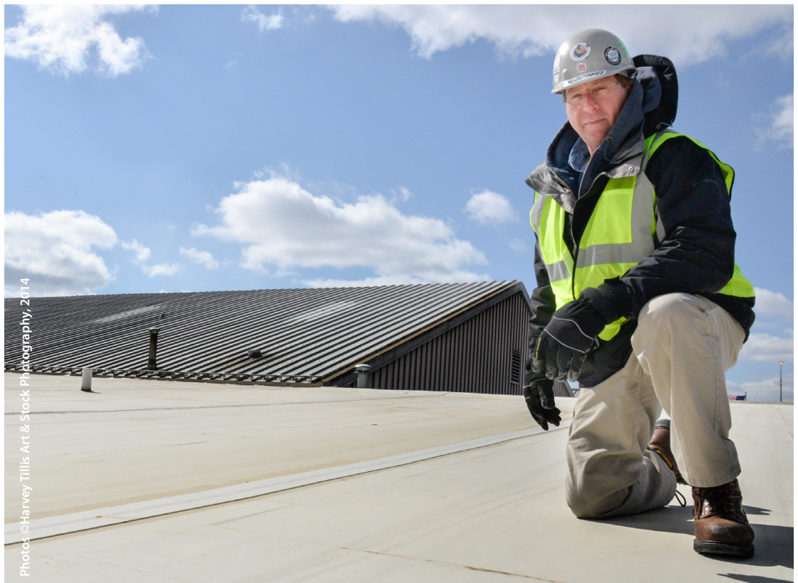
Paul Naretta inspects McDermaid's white roof project at the Marengo maintenance facility along the Jane Addams Memorial Tollway (I-90).
